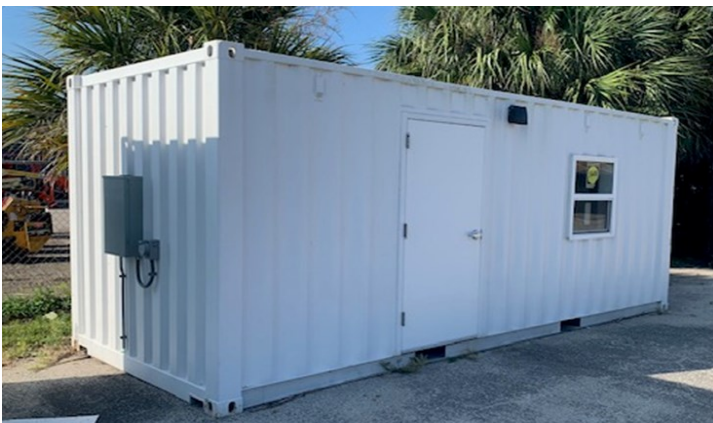
Container/Field Office Bldg for sell. Ready to move..... Can withstand up to 200 mph winds. Constructed by SnapSpace Solutions . Call Jim Cameron 566-2140.
